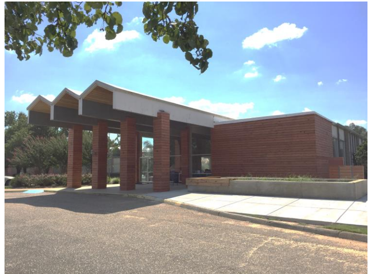
Exterior Façade Update on Front Entrance
